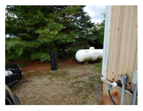
LP gas tank for heating drive-through building and water supply well inside of black plastic pipe.
